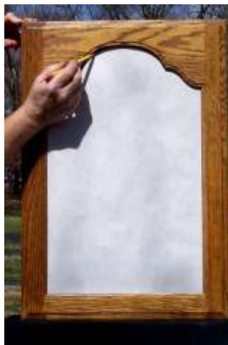
Trace Arch And Inside Door Opening From Front Side Of Door.
